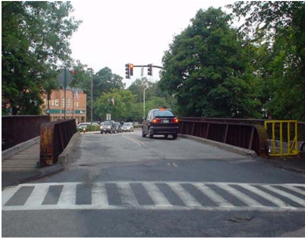
Rockland Street Bridge
